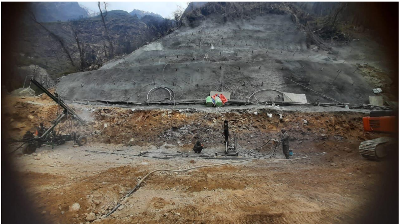
6 Slope Stabilization Work at Mathillo Thulokhola Hydropower Project 22.5 MW
