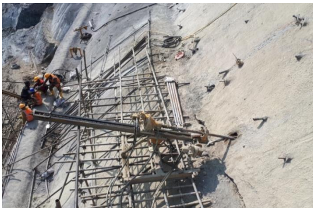
12 mtr Long 76mm dia. Rock Anchoring at Setikhola Hydropower Project (22MW)
