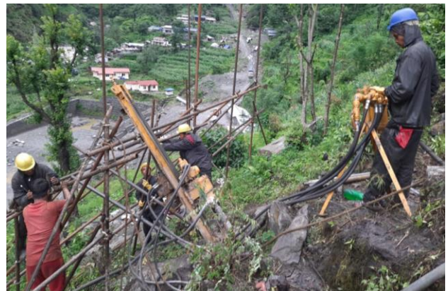
12 mtr Long 76mm dia. Rock Anchoring at Setikhola Hydropower Project (22MW)
