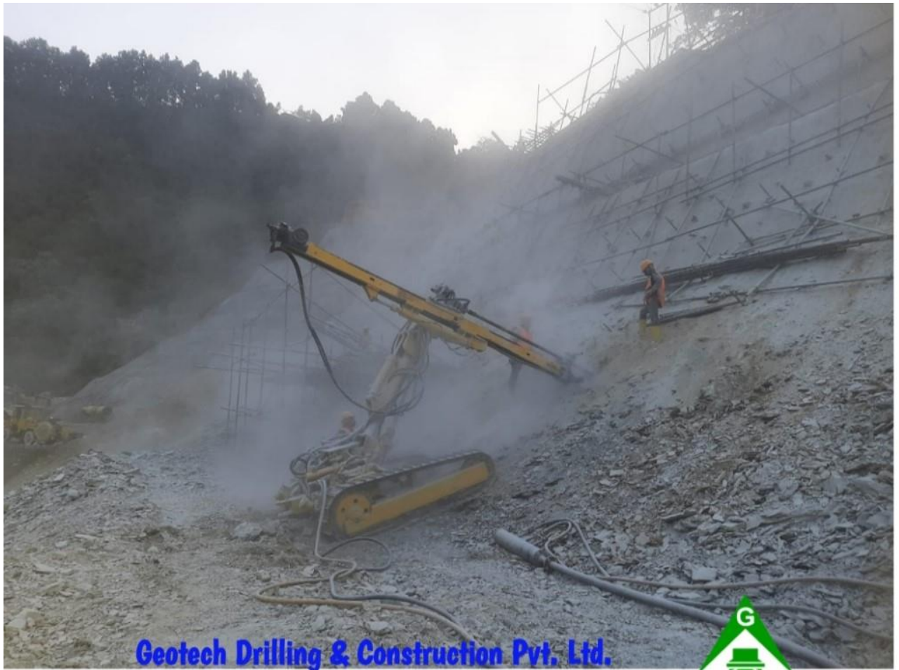
Figure 10 : Rock Anchoring by Crawl Drill for Slope Stabilization work at Setikhola Hydropower Project 22 MW
