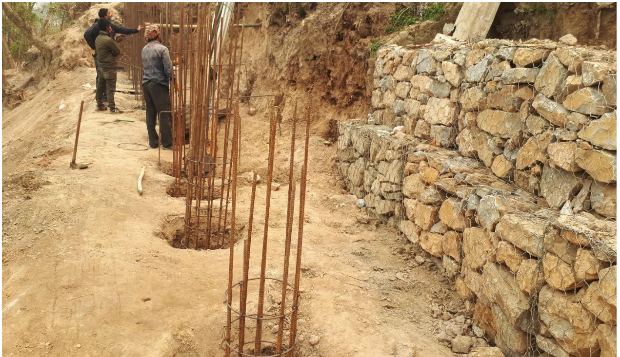
Figure 12: RCC Piling at Kalanki, Under BHU TATHA JALADHAAR NIYANTRAN KAARYAALAYA, Hattiban, Lalitpur
