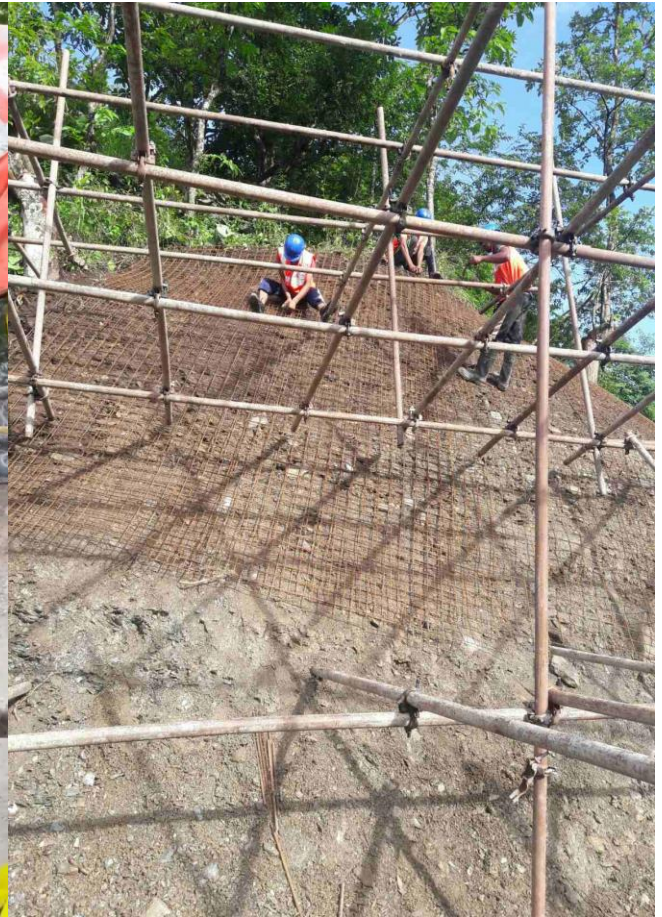
Figure 5: Laying of Wire Mesh before spraying Shotcrete Thulokhola Hydropower Project 22.5 MW
