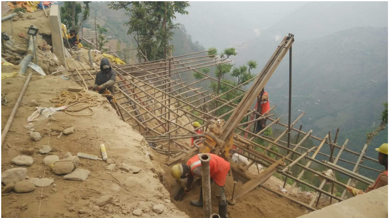
Figure 14 : Micro Piling work at Shree Secondary School, Fikkal, Sindhuli for Slope Stabilization (US aid Project)
