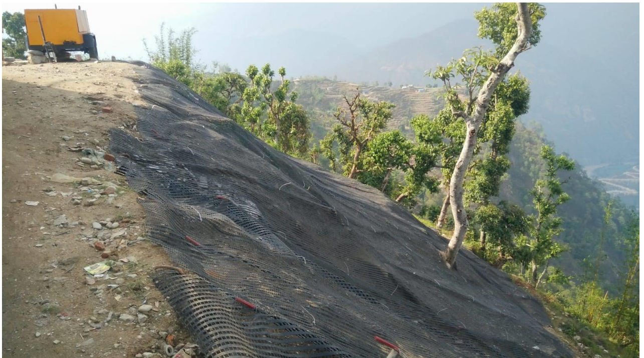
Figure 3 : Laying of Geogrid after completing of Horizontal Micro Pile at Shree Madhyamik Bidhyalaya, Lumti, Sindhuli
