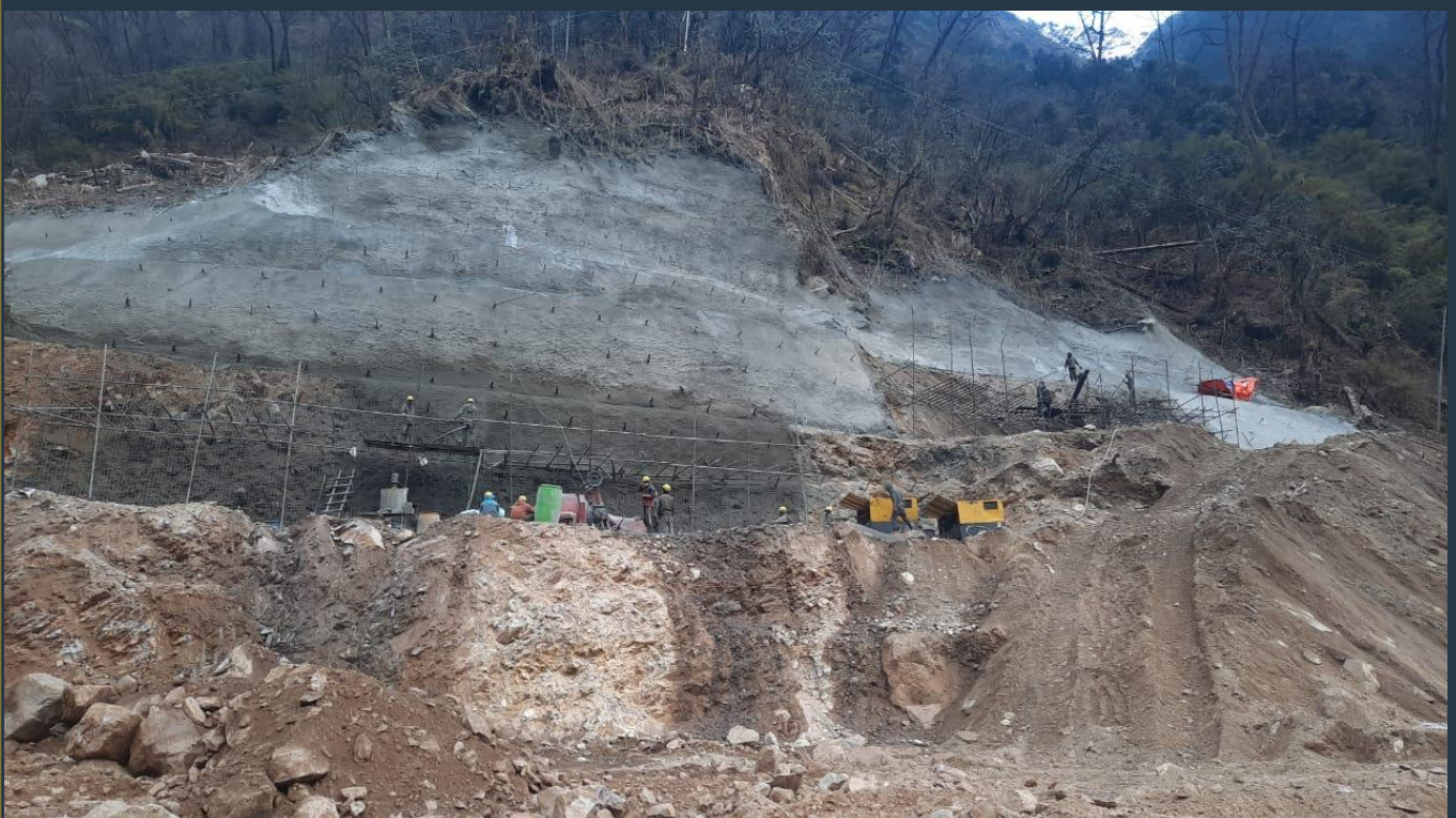
Slope Stabilization Work at Power House of Mathillo Thulphkhola Hydropower Project (22.5MW)
