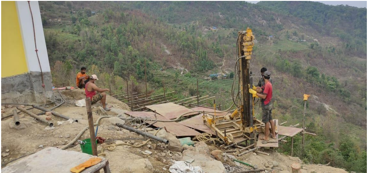
Figure 11 : Vertical Drilling (Micro Piling) at DRSP Project, Sindhuli
