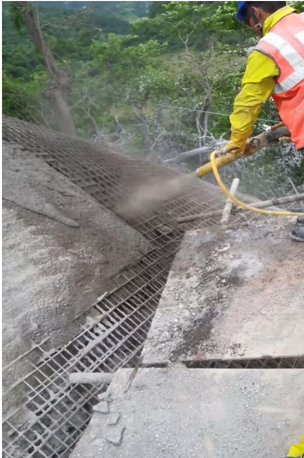
Figure 4 :Spraying of Shotcrete at Mathillo 5 at Mathillo Thulokhola Hydropower Project 22.5 MW
