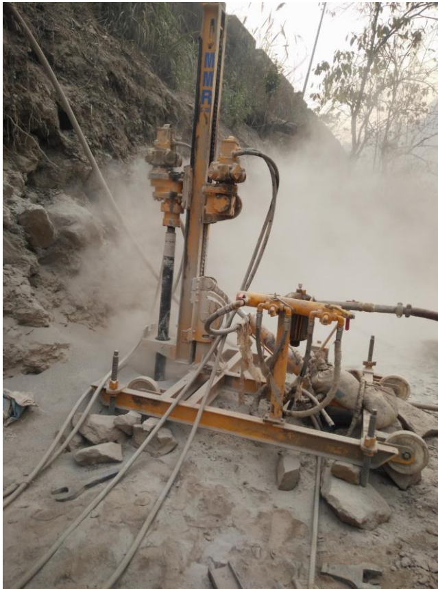
Figure 1 : Vertical Drilling by Skid Mounted DTH at Narayanghat-Muglin Road 17 Kilo
