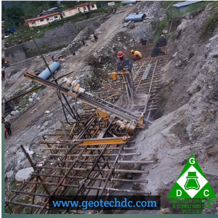
Figure 8 : Rock Anchoring work by DTH at Khanikhola (Dolakha) Hydropower Project 30 MW
