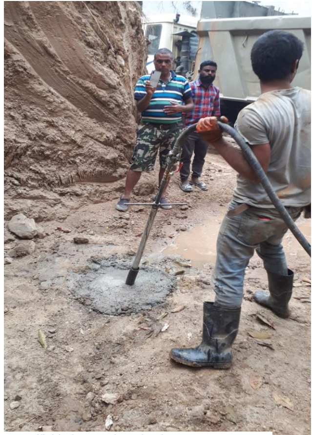
Figure 13 : Drilling & Grouting Work at Landfill Site Bancharedanda
